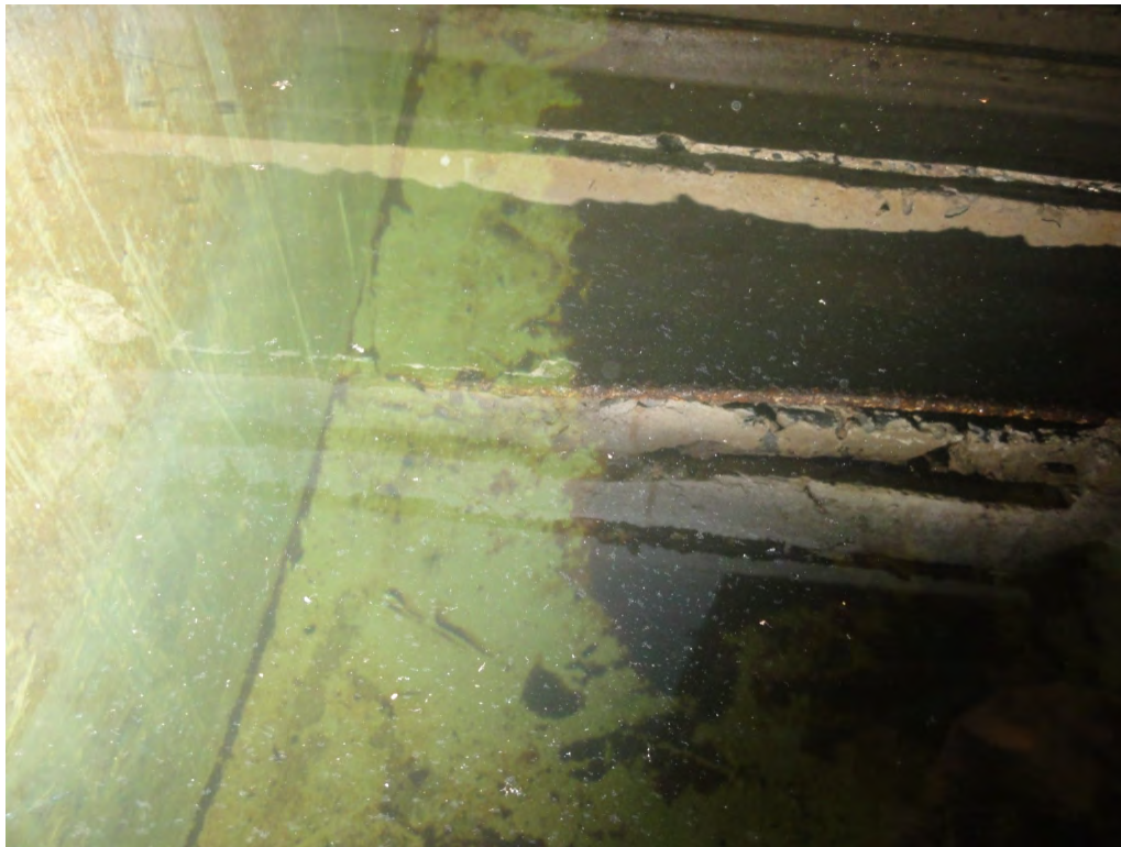
Photograph 28: PH200 – Cistern Photo 1.
