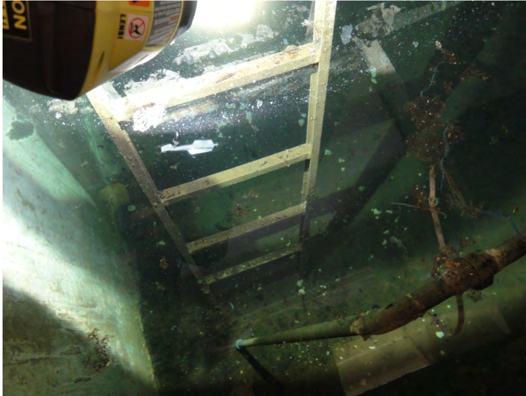
Photograph 21: BV077 – Cistern Photo 1.
