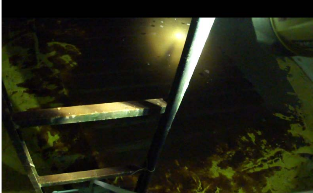
Photograph 27: PH118 – Cistern Photo 2.
