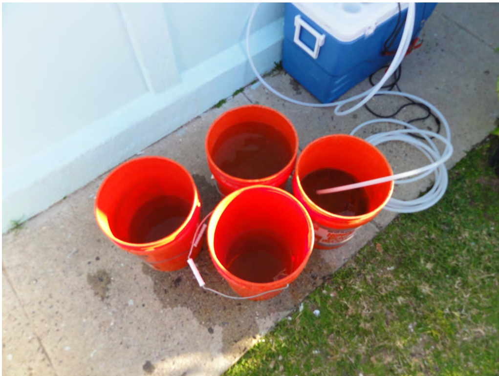
Photograph 32: Sediment vacuumed were discharged to 5-gallon buckets.
