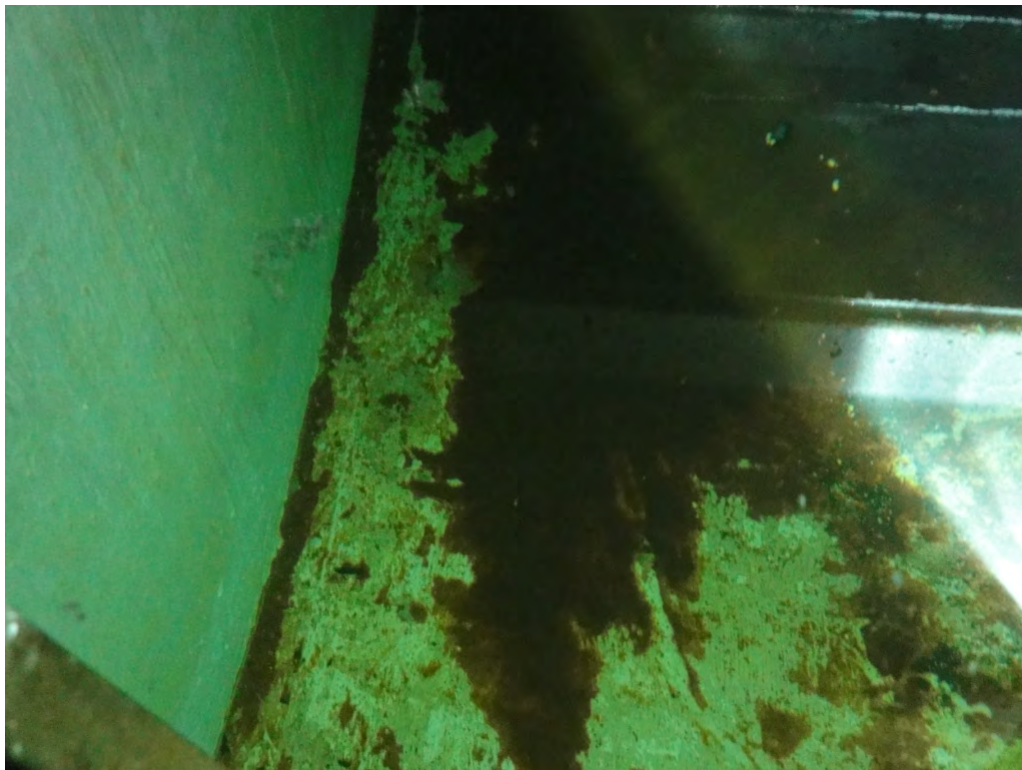
Photograph 24: PH200 - Cistern Photo 1.
