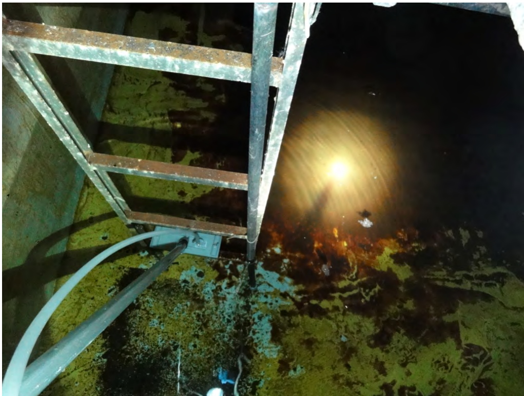
Photograph 26: PH118 – Cistern Photo 1.
